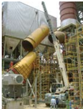
Duct Installation
