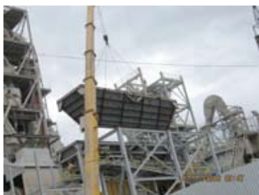
Bag House Second Hopper Being Installed
