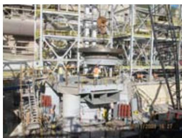
Mill Table Being Installed
