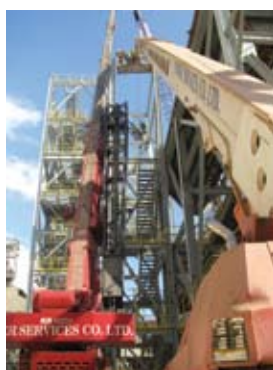
Erection of Feed Tower
